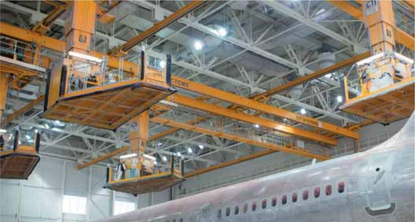
Equipment such as this teleplatform system from CTI Systems of Luxembourg facilitate access to the aircraft within the hangar. The CTI system installed at MNG Technic consists of four bridge cranes and four teleplatform units for painting aircraft up to 777 size.
